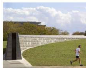
POTOMAC PARK LEVEE, WASHINGTON DC
